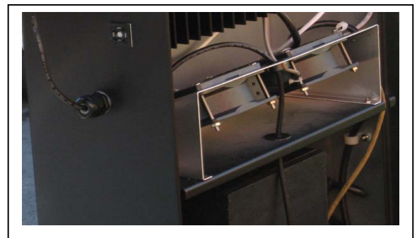
Run wire to bottom area of CODs
